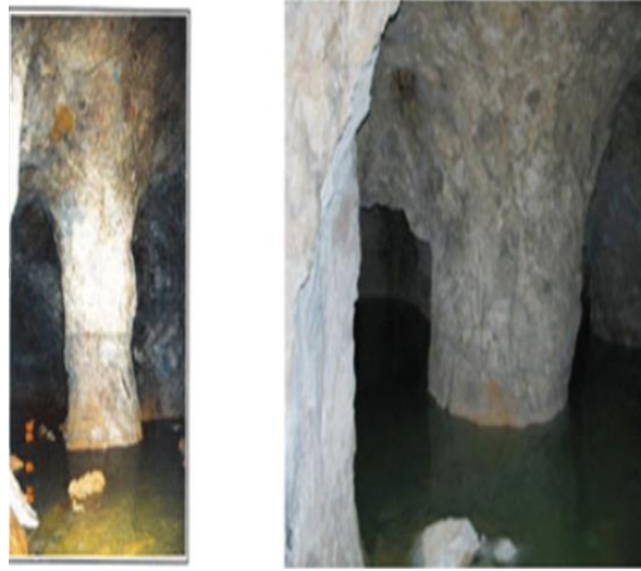
Figure 18. Photo of pillar in the abandoned quarry with a thin layer of water at its base (by courtesy of Watelet JM, INERIS)
