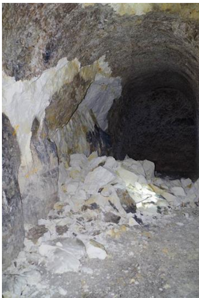
Figure 15. View of the disorders observed after the extreme hydroclimatic event of June 2016, affecting a fault (on the left) and packing down the brickwork through the remobilisation of the embankments at the base of the galleries (on the right)
