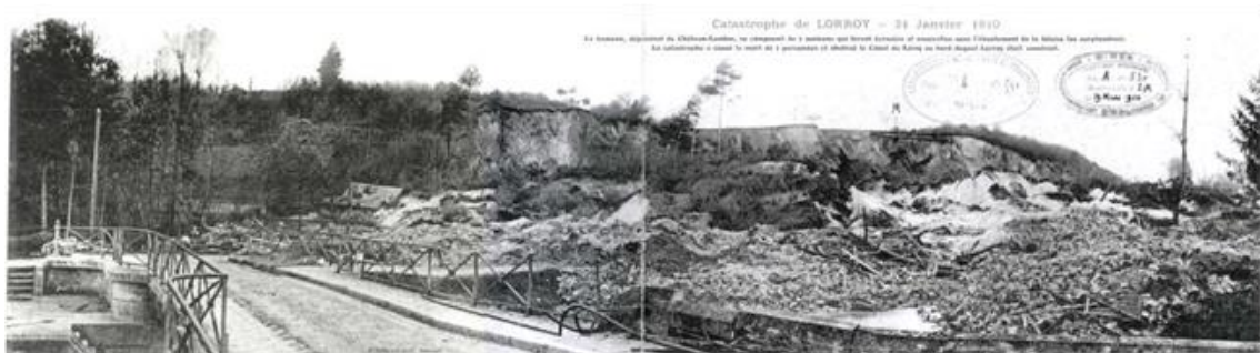
Figure 4. View of the area after the collapse (source: DRIEE IdF archives) The tear-off surface can be seen at the far end.
