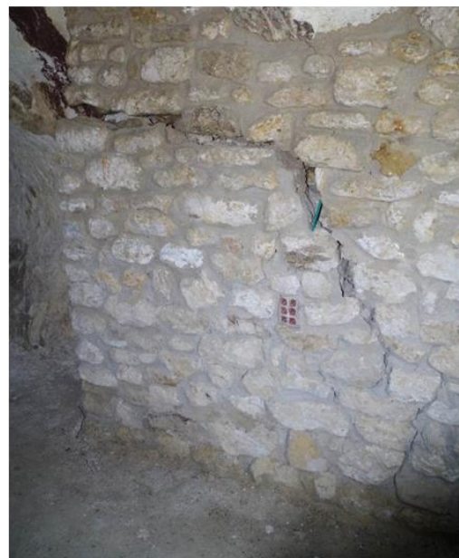
Figure 15. View of the disorders observed after the extreme hydroclimatic event of June 2016, affecting a fault (on the left) and packing down the brickwork through the remobilisation of the embankments at the base of the galleries (on the right)
