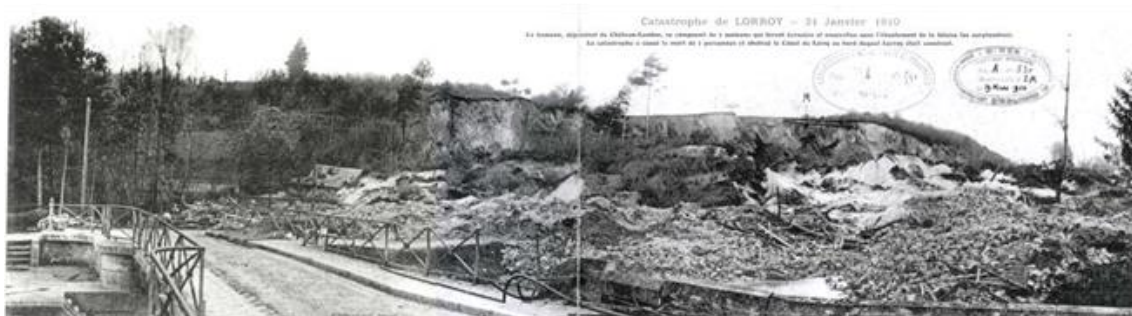
Figure 4. View of the area after the collapse (source: DRIEE IdF archives) The tear-off surface can be seen at the far end.
