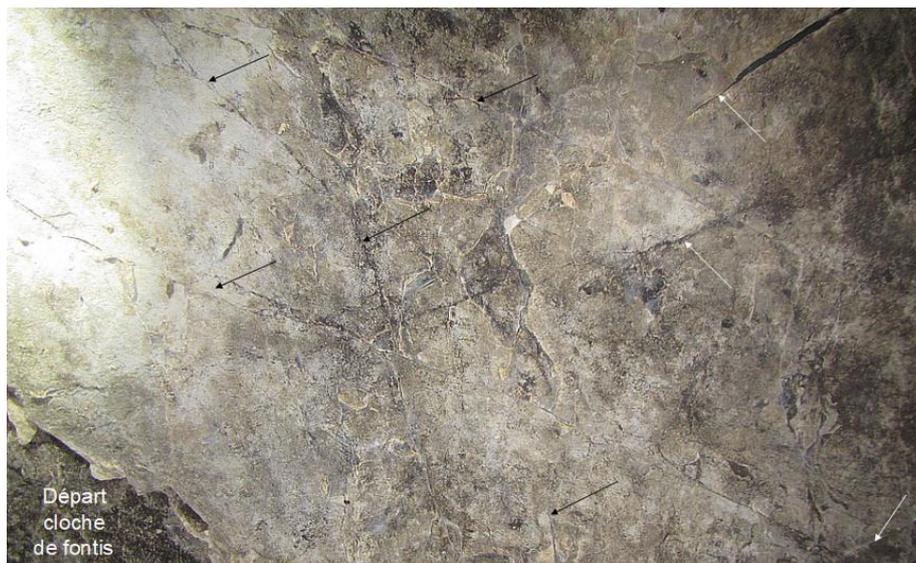
**Figure 13. Photos of the roof of one of the galleries. The multiple conjugate fractures (arrows) testify to the intense fracturing of the galleries (Cerema, 2020).**
