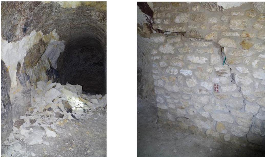
**Figure 15. View of the disorders observed after the extreme hydroclimatic event of June 2016, affecting a fault (on the left) and packing down the brickwork through the remobilisation of the embankments at the base of the galleries (on the right)**
