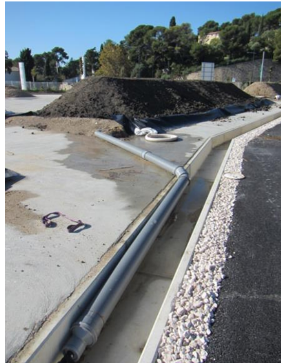
Figure 3: Pilot landform and its percolation collecting system
