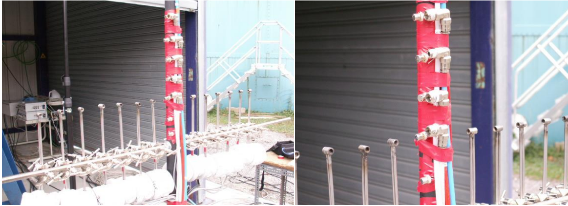
Figure 2 : measurement devices : 11 oxygen sensors and 14 velocity probes (probes developed by INERIS based on McCaffrey probes)
