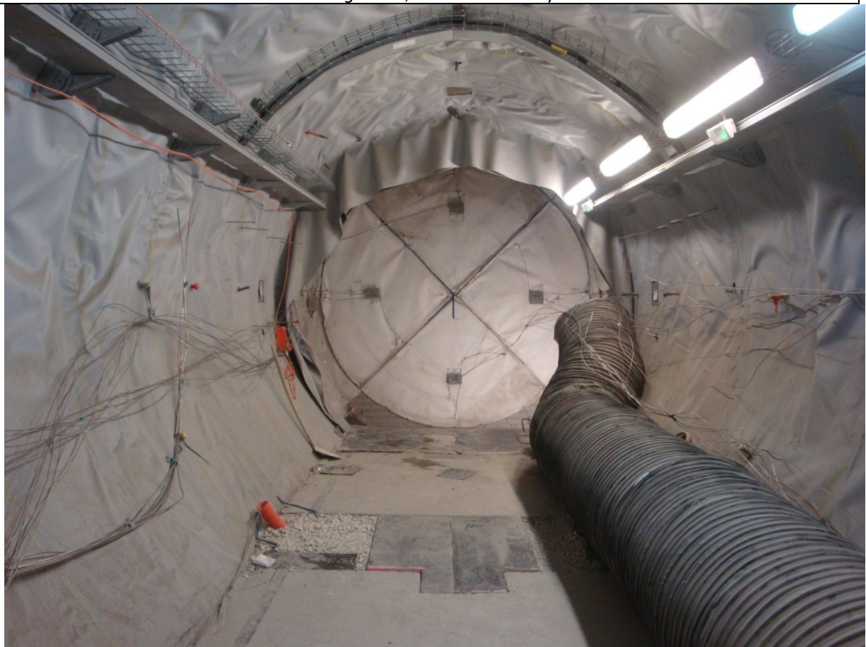
View of the hydration membrane at the interface with the concrete plug (see figure 2)
