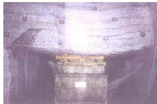
Figure 5: Example of separation of roof (source, MDPA 2015).
