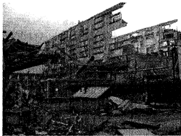
Fig. 1: Destroyed building at a chemical facility.
