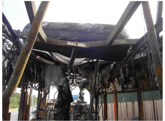
Figure 14: View of tank n°1 that exploded (one half)
