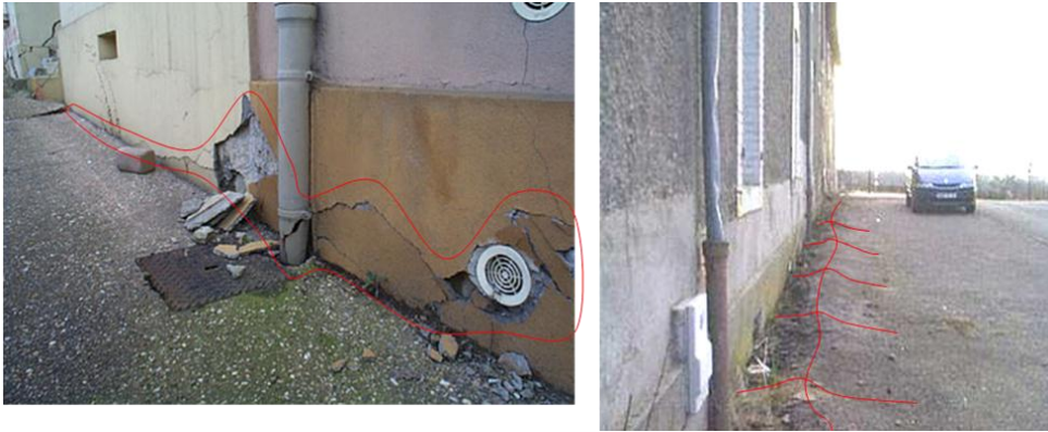
Figure 2: Example of serious structure damages due to subsidence – Iron mine – Lorraine – France
