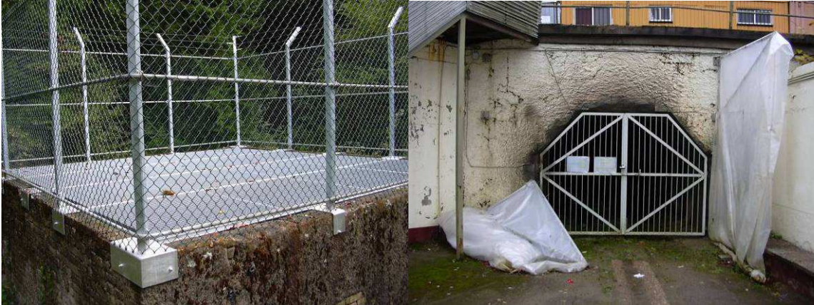
Figure 3: François shaft (left) and Algrange adit (right).
