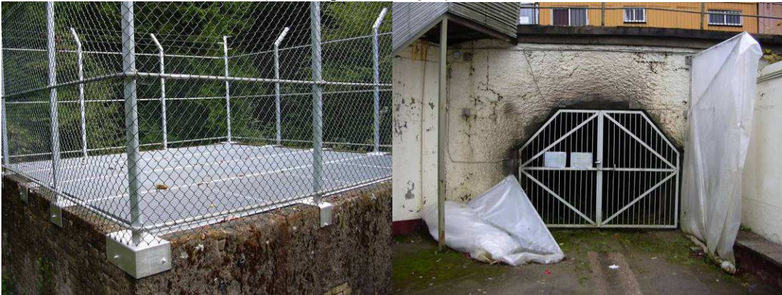
Figure 3: François shaft (left) and Algrange adit (right).
