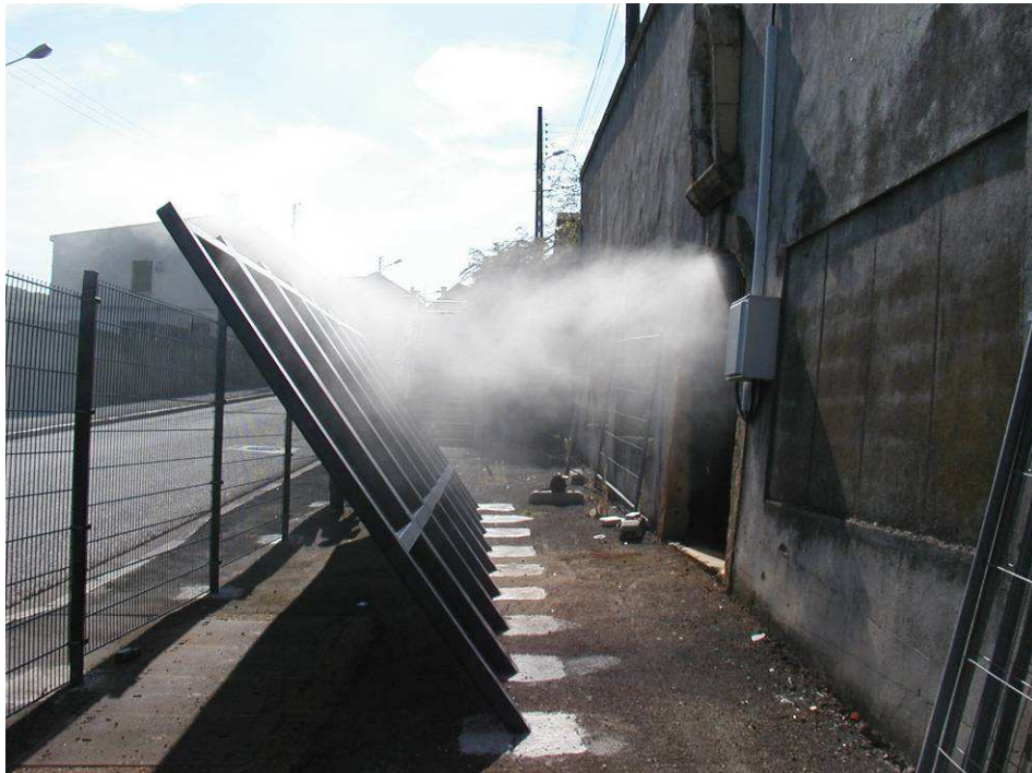
Figure 12: Deflector and enclosure set up at G7 adit exit.
