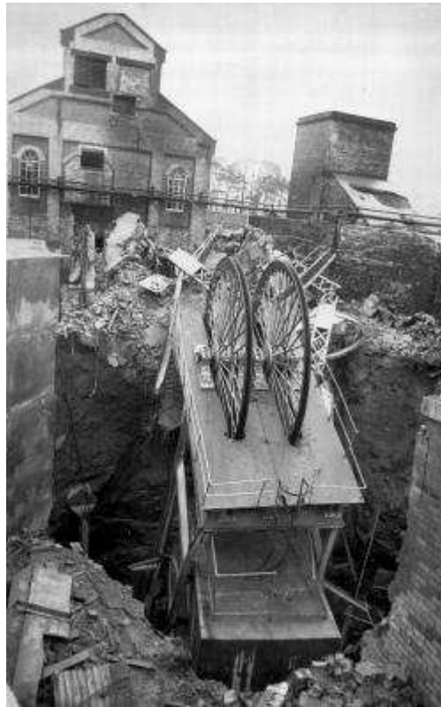
Figure 3 : N°2 Shaft following Collapse (Source: MRSL)
