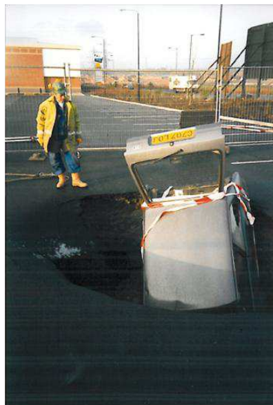
Figure 2 : Collapse of ground in the car park area (Source: UK Coal Authority)
