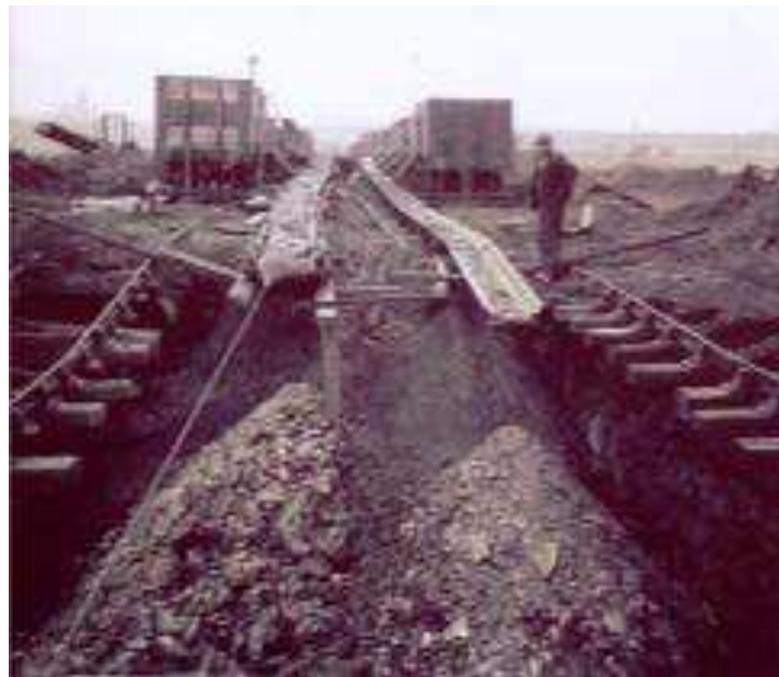
Figure 4 : Infilling Shaft Post Collapse (Source: MRSL)
