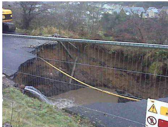
Figure 5: the collapsed shaft at road between Brithdir and Tirphil (Source: UK Coal Authority)
