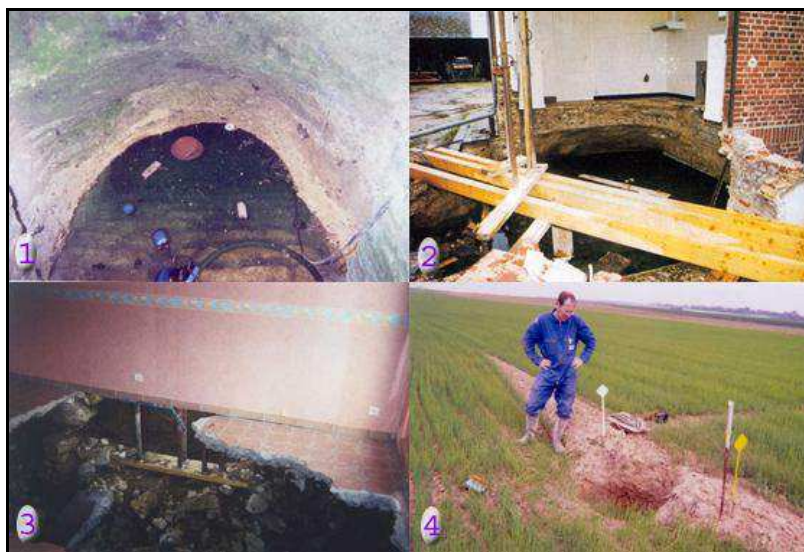
Figure 3: (1) Flooded cellar; (2 & 3) Collapses of buildings due to undermining cavity failure; (4) Backfill run out of an old chalk mine.
