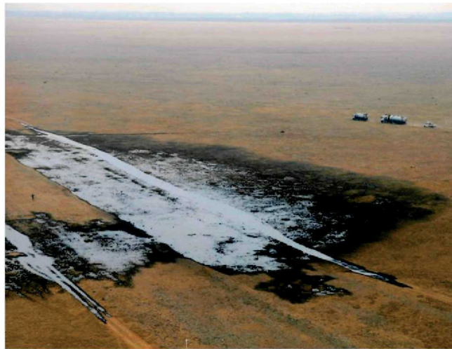
Leak on a crude oil pipeline (Saint-Martin-de-Crau, France, 2009)
