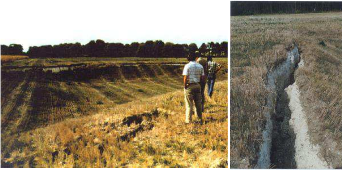
Figure 3: Massive discontinuous subsidence associated with vertical cracks above a French chalk mine.
