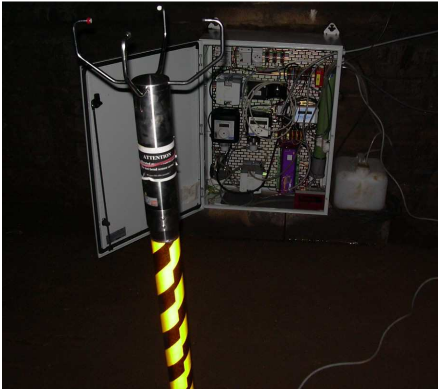
Photo 1. Measuring station and anemometer in Algrange adit
