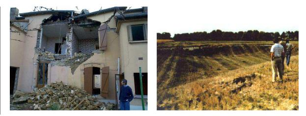
Figure 3. Effect of severe subsidence in Lorraine iron field (left) and major collapse of a chalk mine (right).
