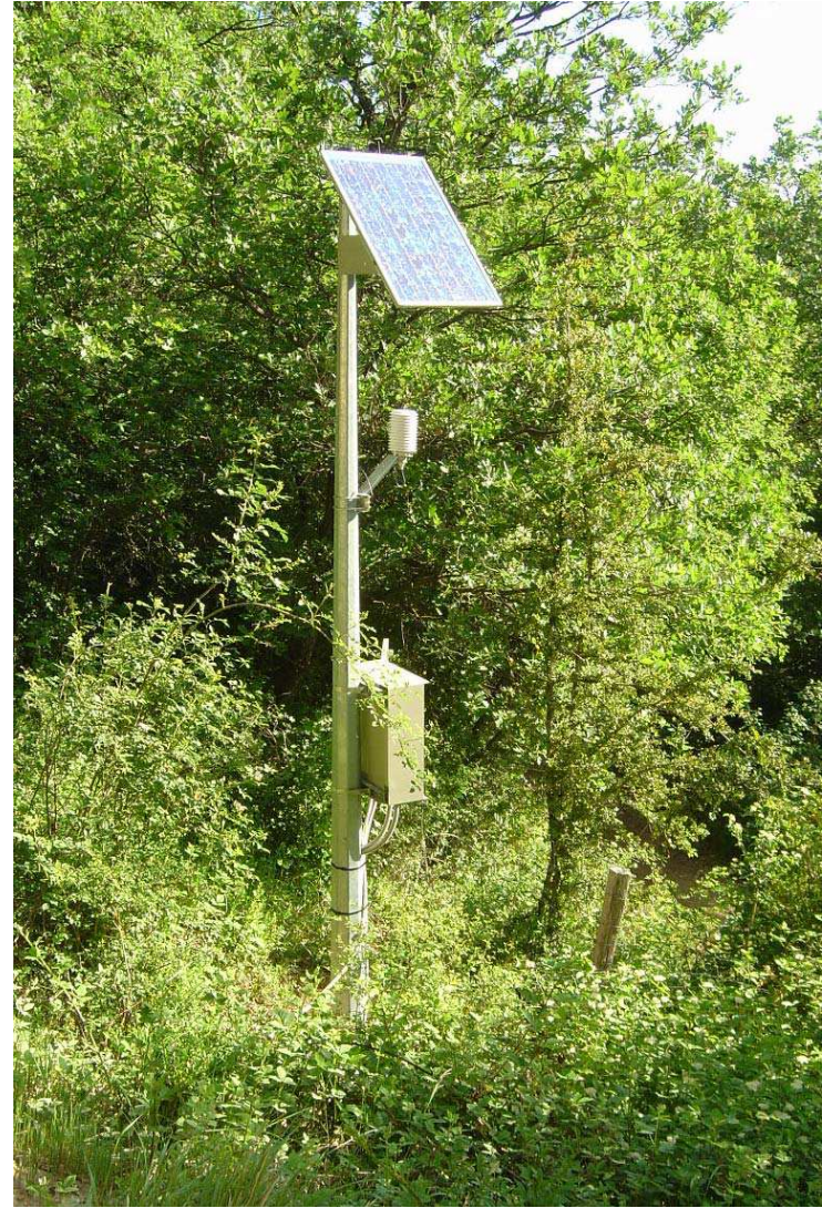
Figure 8. Whole view of the station
