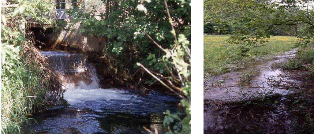
Figure 3. Discharge through an adit (left) and development of a wet zone close to an other adit (right).
