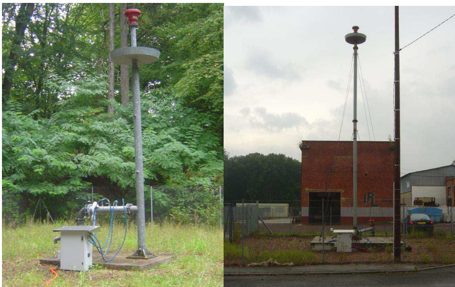
Fig. 1 Photographs of the venting borehole SDEC OUEST 1 (left) and Barrois shaft with a vent (right) (Lorraine coal basin)
