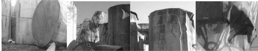
Figure 1. (a) Knocking over of a tank (b) Deflection of two slender tank (c) Global buckling (d) Local deformation (Mouilleau et al., 2001)
